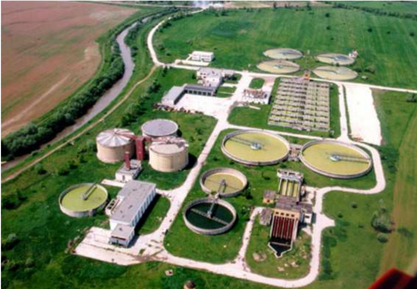
NATO's Sarajevo WWTP
