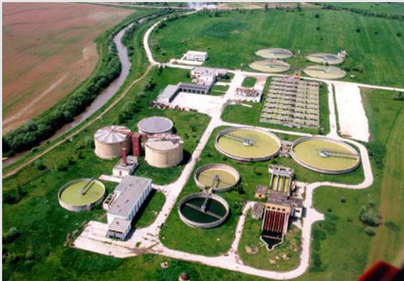
NATO's Sarajevo WWTP
