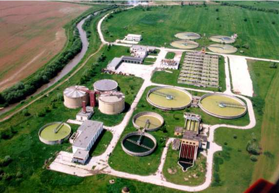
NATO's Sarajevo WWTP
