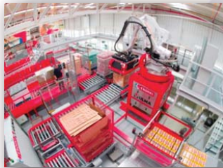
Automated Warehouse (AW) ULMA Handling Systems, Spain
