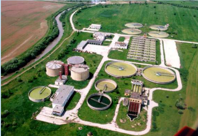
NATO's Sarajevo Waste Water Treatment Plant
