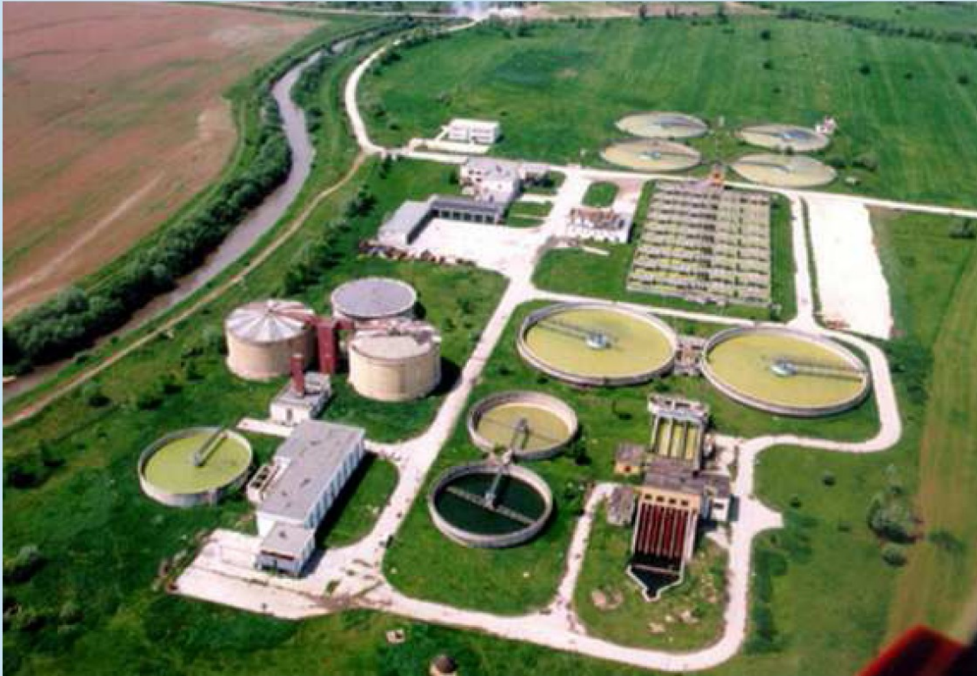
NATO's Sarajevo Waste Water Treatment Plant
