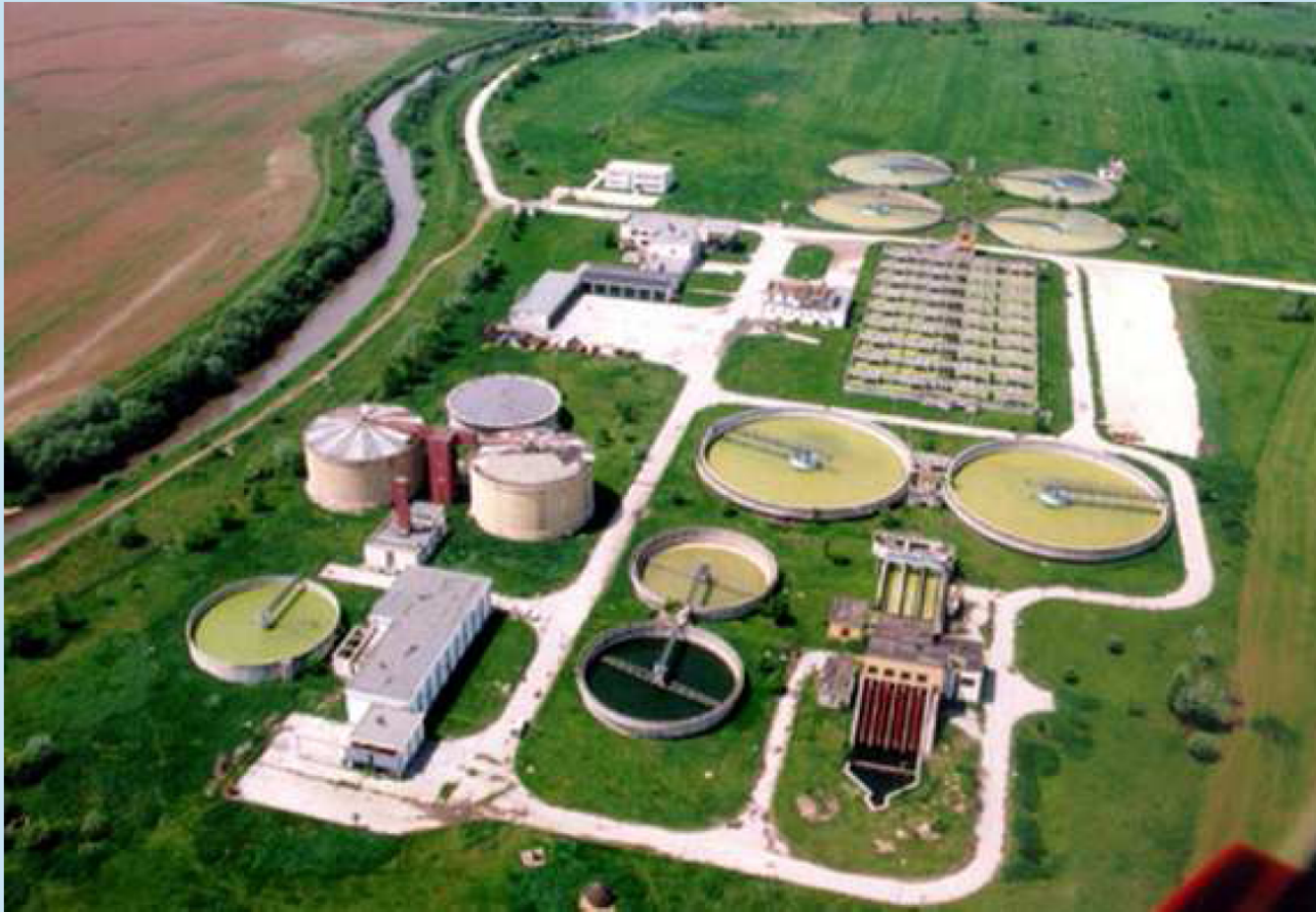
NATO's Sarajevo Waste Water Treatment Plant
