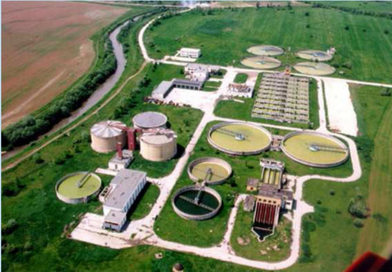
NATO's Sarajevo Waste Water Treatment Plant
